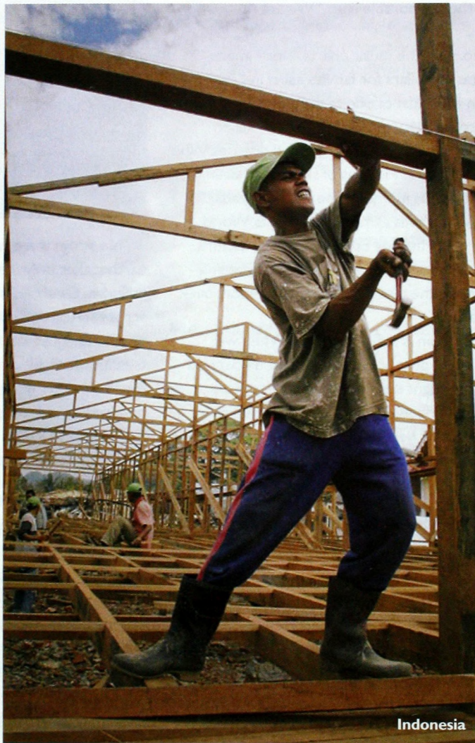
Rebuilding is under way in tsunami-devastated Indonesia.
